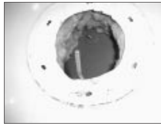
The temperature probe installed on a tank.
